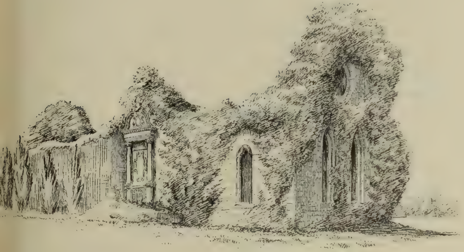
FIG. 1412.—Keith Church. View from South-East.
